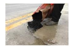
Perma-Patch® is a completely new type of paving material developed to fulfill a need to rapidly, safely, and permanently repair potholes, utility cuts, T.V. or fiber optic cable slots, and parking area problems in all types of weather.
